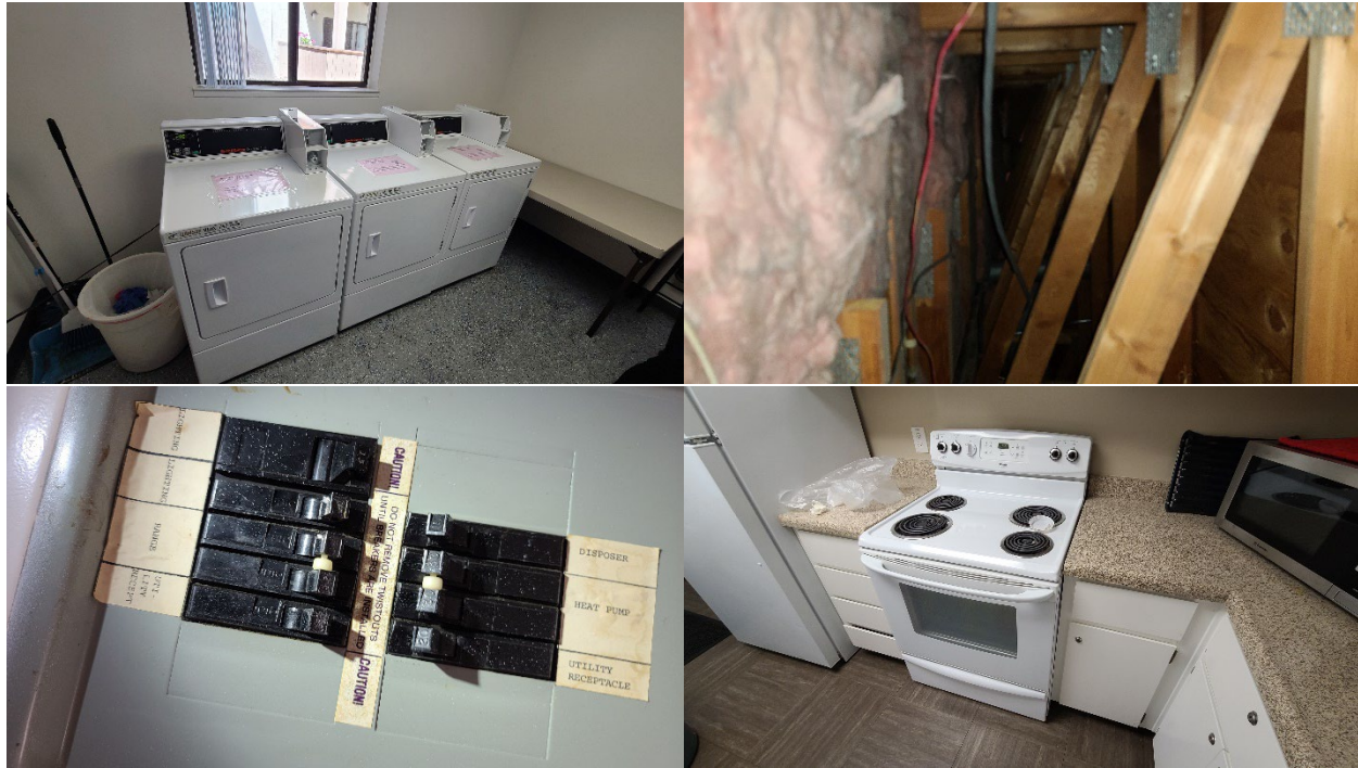
Top row, left to right: forced air rooftop packaged unit and available space on flat roof. Second row, left to right: 600A building main breaker and main breaker to units. Third row, left to right: meter bank and central DHW. Fourth row, left to right: gas-fired clothes dryers in common area laundry and existing attic insulation (rotated). Fifth (bottom) row, left to right: apartment unit breaker panel and in-unit electric cooking range.
