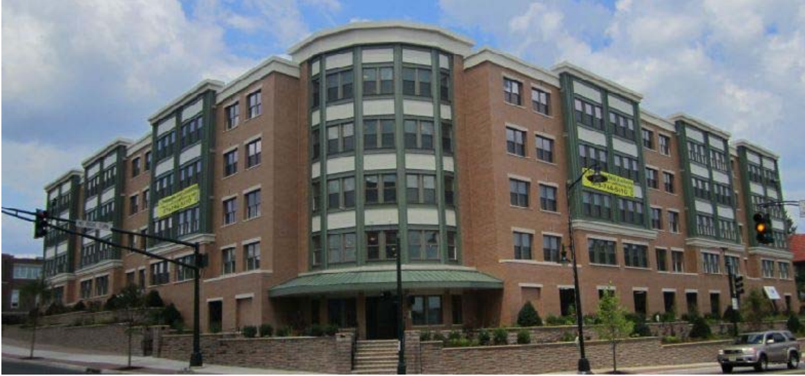
Figure 30: NJCC5 - NJCC11 Multifamily Building Photo, RPM Development
